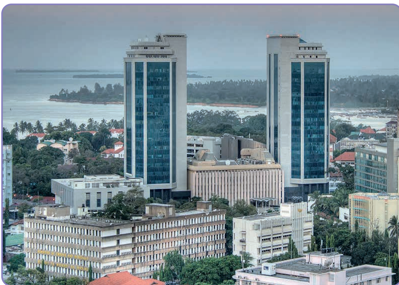
Bank of Tanzania – Sub Head Office, Dar es Salaam (Photo: BOT Website)
